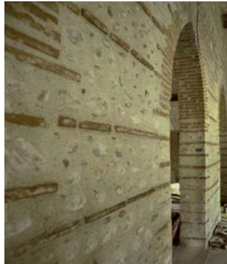
Historic internal wall repaired with Natural Hydraulic Lime mortar
